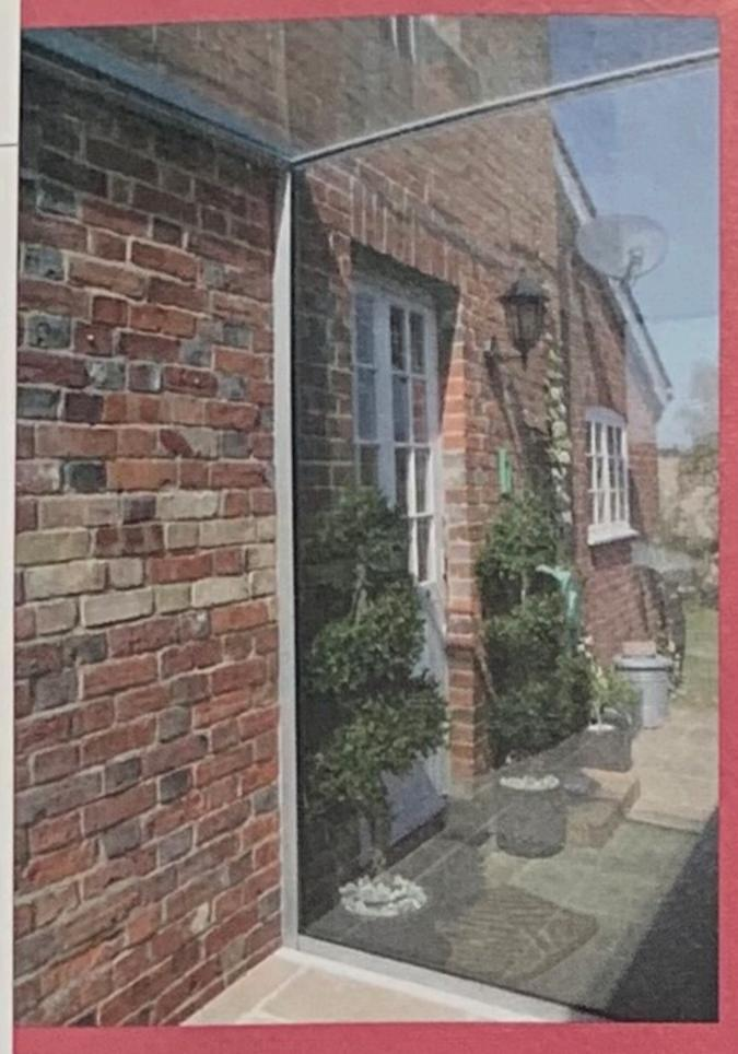
Ion Glass was commissioned to create a fully bespoke structural glass link in this listed oast house to connect the newly built dining and entertainment area to the kitchen in the original building. Made from clear laminated glass the panels are double-glazed for full heat insulation, ensuring the link is fully compliant with Building Regulations and heat loss regulations. The glass wall and roof panels were individually manufactured to fit precisely within the space.
